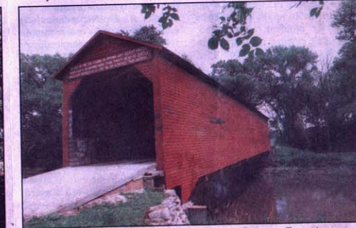
The Oquawka Wagon Bridge in Henderson County was built in 1866 and served the area for 68 years. (Photo by Tony Miller)
