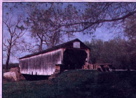
Mary's River Covered Bridge in Randolph County was built in 1854, restored in 1954. It rests on original stone abutments. (Photo by Gene Howard, "Covered Bridges of the Midwest")
